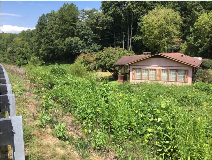
Site 10 Photo Point #1 (Downstream)
